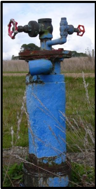
This is Bore 82840 at Wire Lane before it was reconditioned sometime between 2010 and 2012. The Top Of Casing (TOC) was approximately 900mm above groundlevel.
